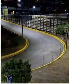
England Jordan Highway Project
